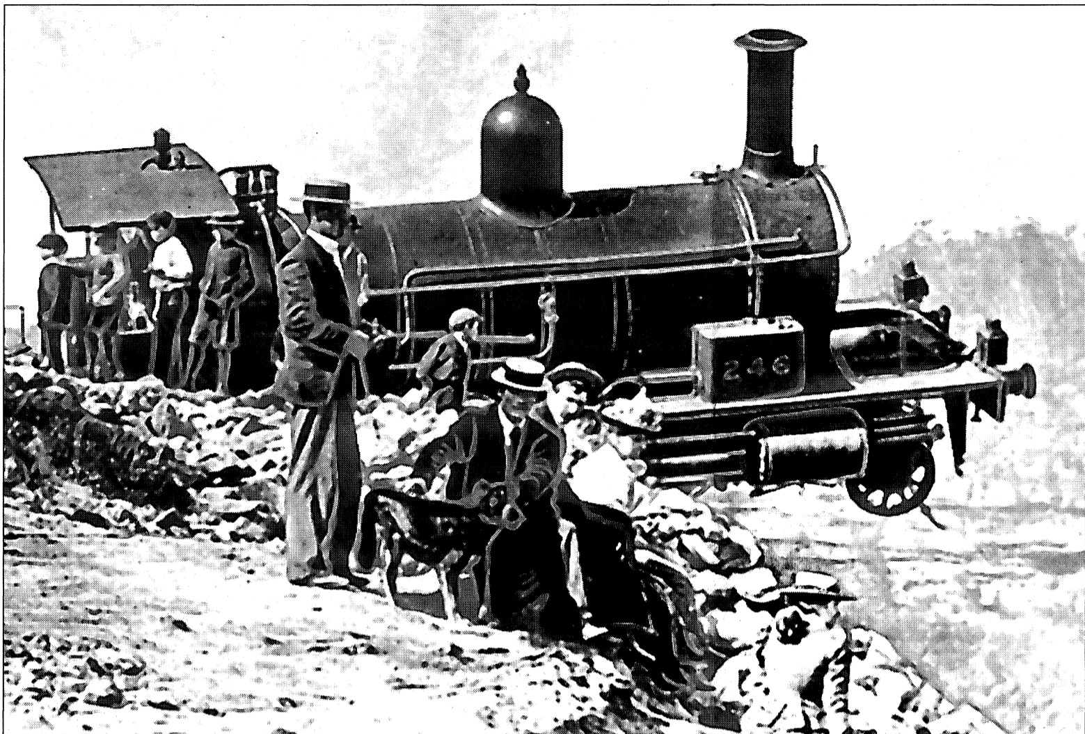
Locomotive B246 came to grief in 1910 on the Zig Zag Railway after a brake failure in the Blue Mountains. The driver and fireman managed to leap clear of the dangling engine and nobody was hurt. But 83 died and 213 were injured in the nation's worst rail accident (below) at Granville, Sydney, in 1977.
