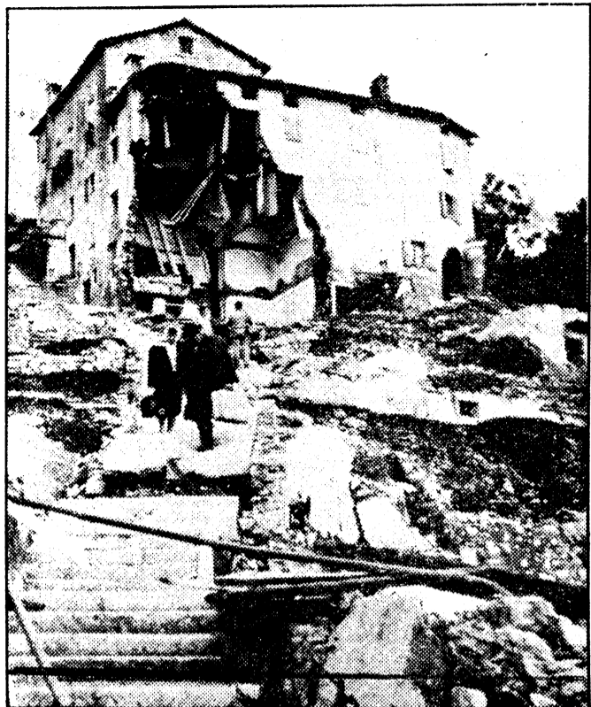
This house was partially destroyed by the water's fury but rendered unliveable. The inhabitants later rescued their few remaining possessions.
