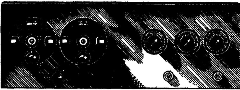
**The front panel of an 8-valve build-it-yourself superhet described in 'Wireless Weekly' for July 29, 1927. The main controls are (L to R) oscillator tuning, loop aerial tuning, IF amplifier filament current and bias, and detector filament current.**
