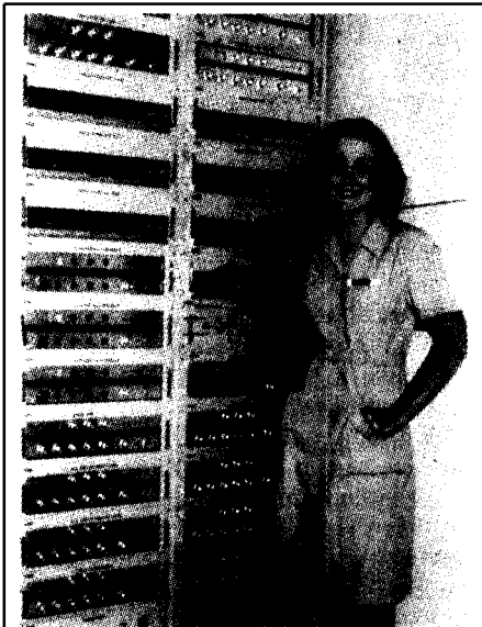
Fig.4: A Nomis communications system produced for the Adelaide Children's hospital. It provided bedside music, radio, TV sound, paging and intercommunication for the hospital proper and associated nursing homes.
