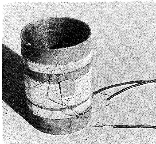
**This hand-wound coil, along with the screw-assembled cabinet, the simple 3-valve format, and no maker's nameplate, gave the impression that the regenerative radio was sold in kit form. Build your own was a popular concept in the 1920s.**
