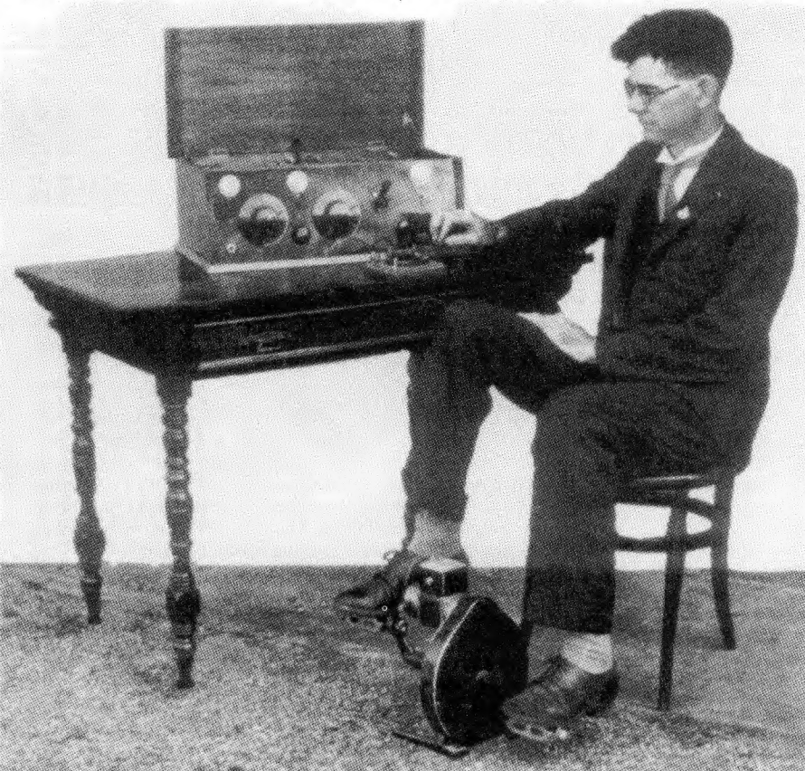
Alfred Traeger posing with the first pedal radio in November 1928. This consisted of a 2-valve regenerative receiver using space charge tetrode valves (A141) and a 1-valve triode (B205) crystal-controlled Morse code (CW) transmitter. The transmitter operated with an output of 1-1.5W on a frequency of 2230kHz.
