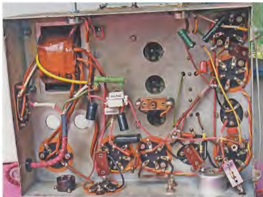
Most of the carbon resistors and all the paper capacitors were faulty and had to be replaced, along with the electrolytic filter capacitors. The wiring to the mains output socket at bottom left was disconnected in the interests of safety.
