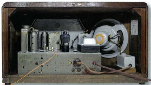
The two HT electrolytic filter capacitors are located in a box that's spliced into the speaker cable. These capacitors had previously been replaced, as had electrolytic capacitors C11 & C29.
