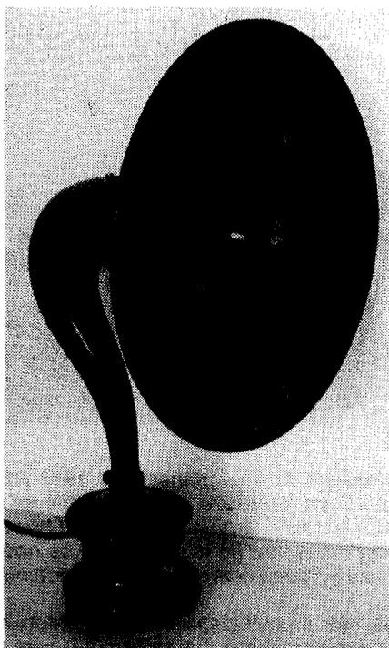
*A skilled panelbeater, a spray painter and an artist all contributed to the restoration of this Claritone speaker. Originally, the flare had a hole in it from being nailed to a beam, and much of the paint was missing. After the metal repairs, the horn was resprayed in black cellulose lacquer and the logo was repainted from a photograph. Not a project for the novice!*
