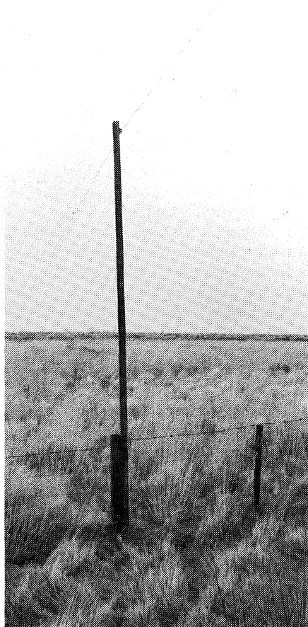
Fig.3: The Southland Branch of the New Zealand DX League has a listening post with a selection of Beverage aerials providing world-wide reception of MF transmissions. Situated on a tussock and scrub covered shingle spit with sea water on practically three sides, and with the nearest power line a couple of kilometres distant, conditions are ideal for this type of aerial. This is a typical aerial pole for the Southland array.
