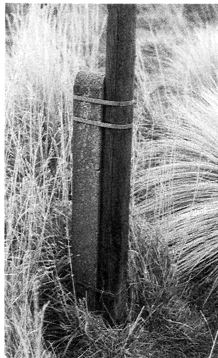
Fig.4: Fence posts can provide secure mountings for lightweight poles, as this close-up shows.
