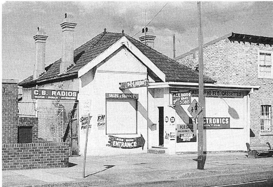
The A.C.E. Radio premises in Marrickville, just before the building was sold. When formed in 1934, the company was registered as Excelair Radio and supplied built-up radio chassis.
