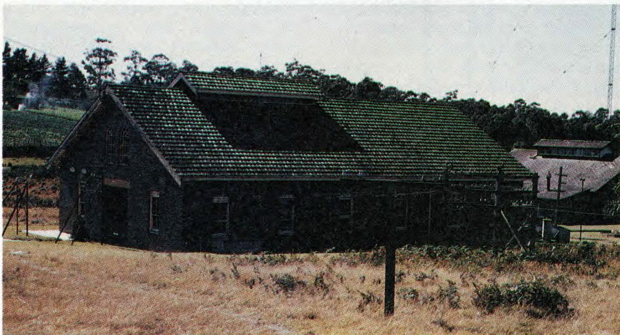
More spacious and better ventilated than the old Telefunken cottage, the 'new' transmitter building accommodated the transmitters around the walls, with control and switching facilities in a centre aisle. At this stage, the facilities were manned 24 hours per day.
