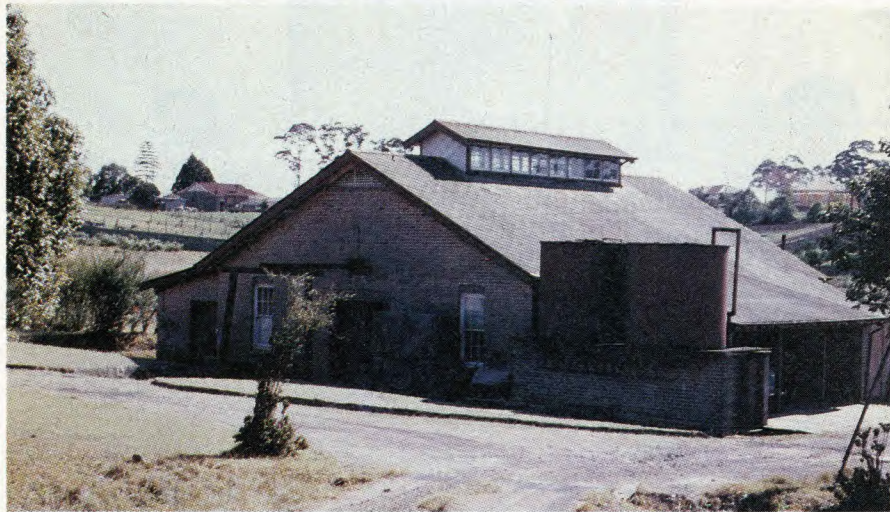
The Engine Room, intended to keep the station on air in the event of a mains failure. Gerry Stanley says that the much patched leather driving belt indicated plenty of work in other days, but he could not remember it ever having been run while he lived in the station.
